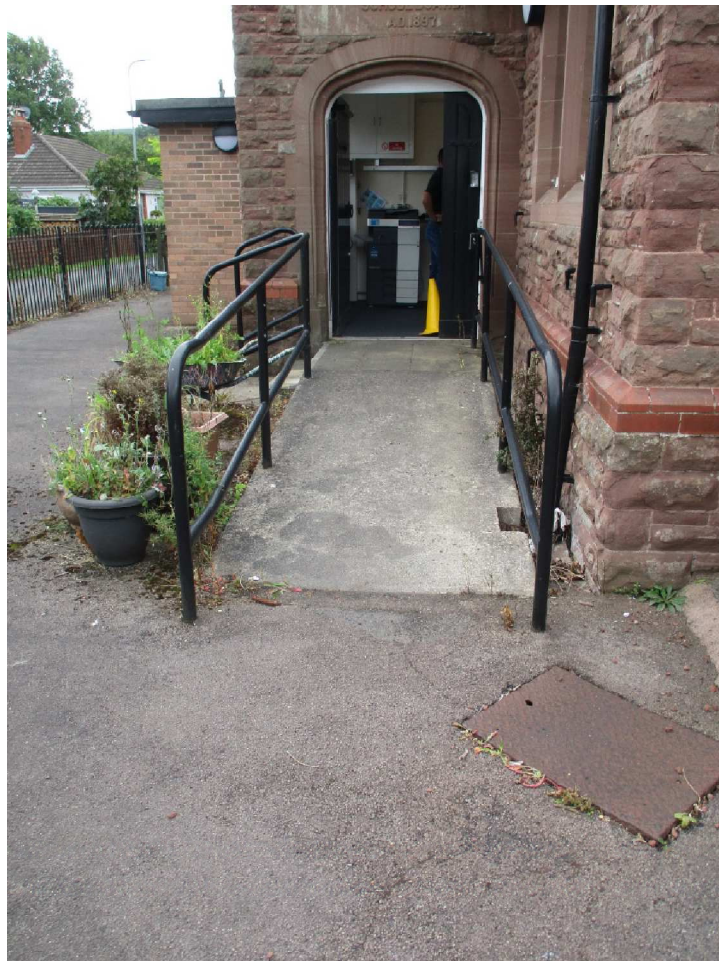
Photo 15 – Entrance ramp/ steps
