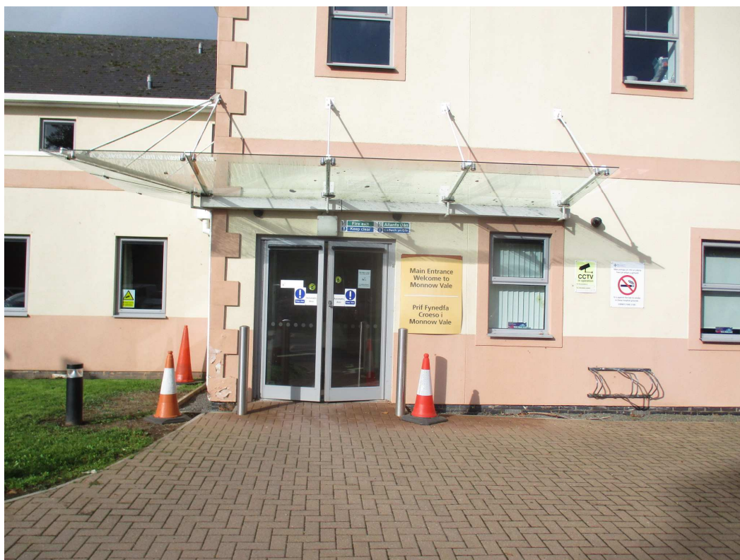
Photo 27 Level entrance/ automatic entrance doors.
